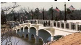
2003-2004, Home Rd. Bridge Replacement Project
