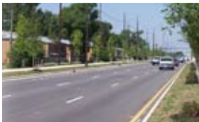
2006-2007, Morse Road Improvements Project
