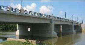
2005-2006, Woody Hayes Bridge Project
