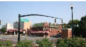
2004-2005, Lane Ave. Widening Project
