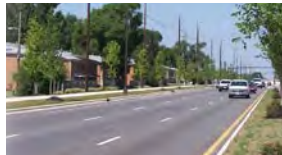
2006-2007, Morse Road Improvement Project
