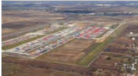
2007-2008, Rickenbacker Intermodal Facility Project
